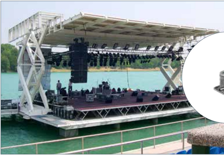
Optimized worm gear screw jacks from Pfaff-silberblau lift and lower the roof of Milan's stage reliably and, above all, safely.
