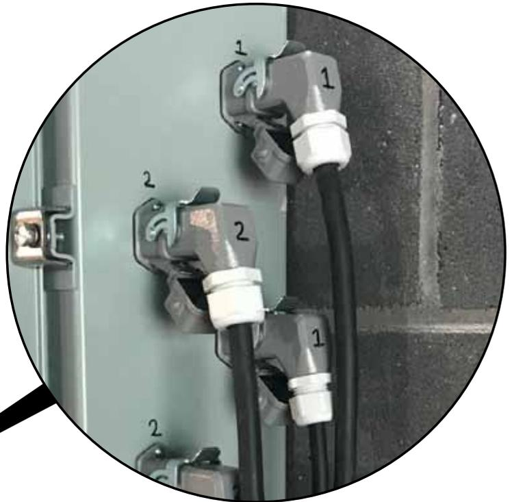
*Actuator motors, limit switches, and encoders designed with quick disconnects at the controls enclosure to be quickly removed and installed to accommodate scheduled maintenance needs.*
